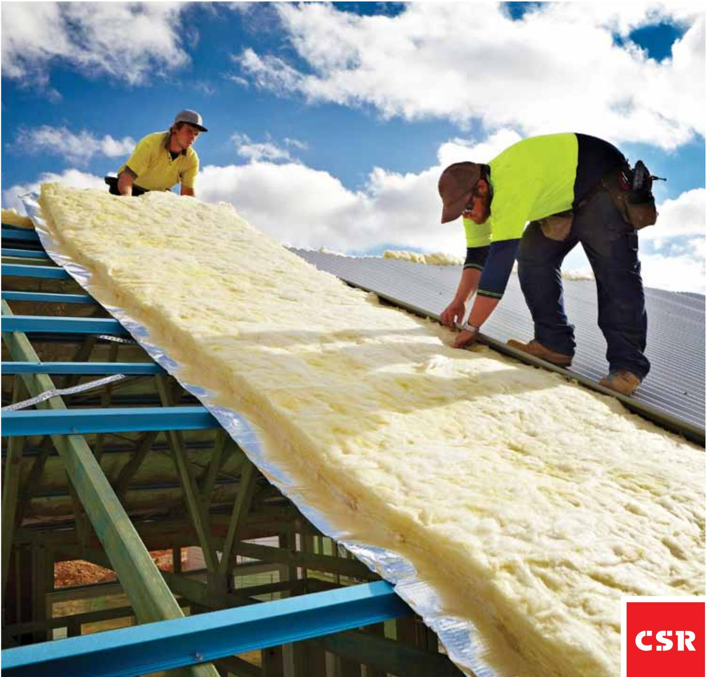
Insulation is proven to be one of the most effective ways of controlling temperature and reducing unwanted noise. Bradford Anticon combines two very effective forms of insulation into a single product to provide these benefits. The reflective foil acts as a barrier, which reduces the radiant heat entering the roof space by up to 97% and also controls condensation, while the insulation blanket absorbs outside noise and dramatically slows the transfer of heat into and out of your home.
